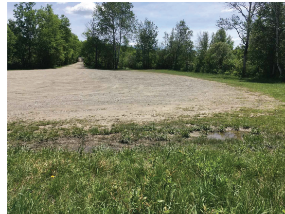
Parking lot runoff collects on the edge of the gravel parking lot. Proposed location of southern bioretention basin.
